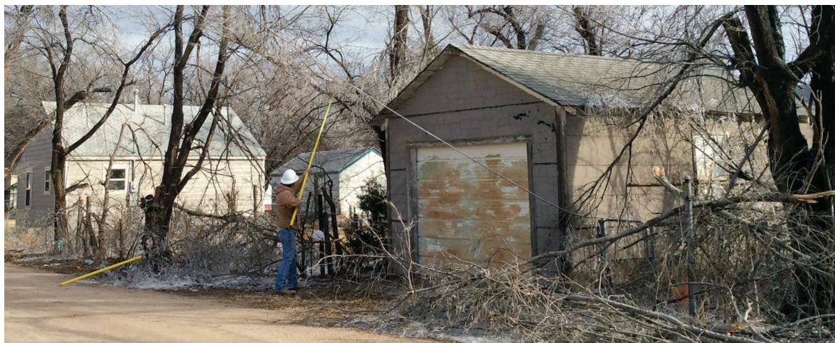
Second year apprentice lineman Jesus Villegas works to clear fallen tree branches from Wheatland lines behind a member's home in Great Bend.
